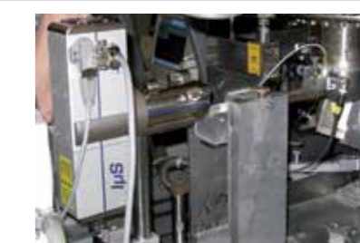
replacement of an old 18 kW Siemens RAG, Halle
